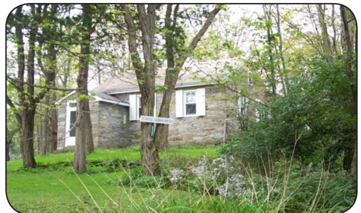
The "House with a Past" in Benson, Vermont
