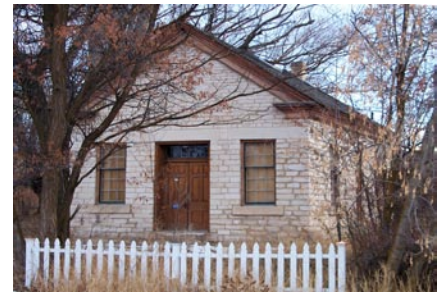
Building in Spring City, Utah purported to be an Endowment House used by Apostle Orson Hyde.
