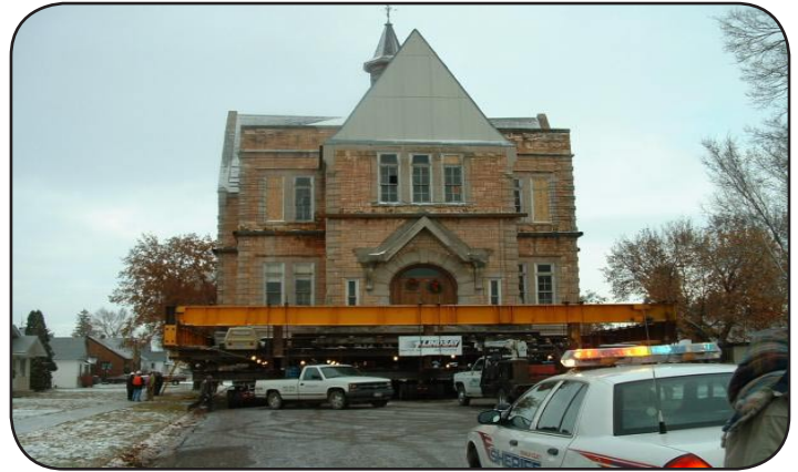
Oneida Academy, Preston, Idaho moving to its new location
